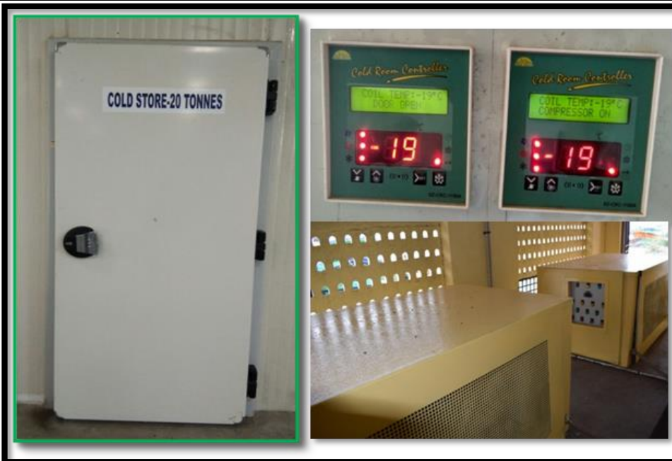
Cold Storage Facility
